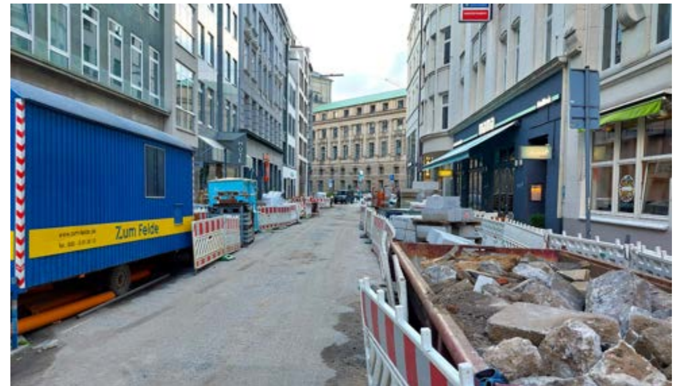
Pavement development in BID Nikolai Quartier
